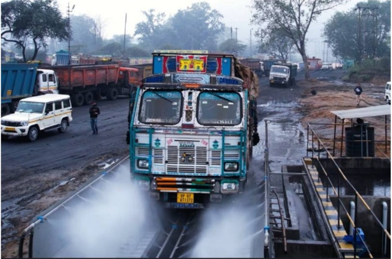
Wheel washing facility at Mine Barrier
